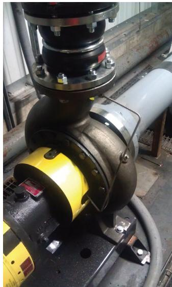
These Gusher ANSI pumps were sold to and installed at Yamaha in Newnan, Georgia. Their service is paint sludge system recirculation. They replaced vertical mount pumps. The pumps are primed via use of a foot valve. Flexaseal single stationary bellows cartridge mounted mechanical seals were installed by Gusher factory with Plan 11 discharge recirculation piping to promote flow in the seal chamber.
