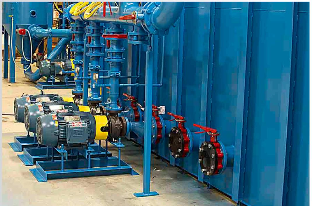
These Gushers are running on an aerospace fastener manufacturer in Southern California. The application is Centerless Grinding- Titanium, Stainless steel fasteners. This is a system to consolidate up to 80 grinding machines into a central system capable of filtering at a rate of 500 GPM of straight oil to a level of clarity below 5 micron. The system has a Gusher filter pump controlled with a VFD along with (3) clean pumps, (two operating with one standby) also utilizing VFD controls.
